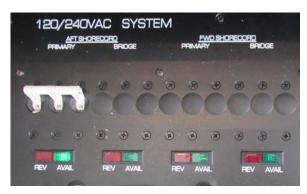
Shore power and generator indicator lights, on the AC distribution panel
