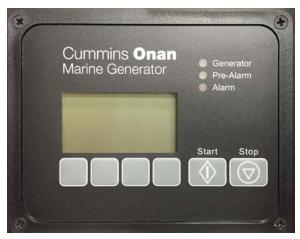
Remote generator control panel, in the starboard galley electrical cabinet
