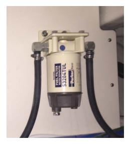
Generator water-separator fuel filter
