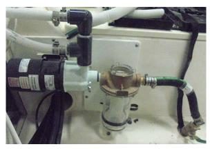
Typical air conditioning pump, strainer, and valve, in the engine room
