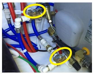
Figure 6-3: Water heater valves in bypass position
