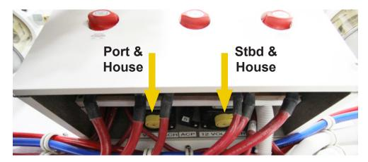
Figure 4-5: Yellow ACR control knobs under Master DC Panel
