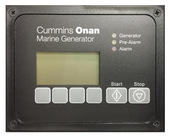
Figure 5-8: Generator control panel,in the port storage cabinet in the atrium
