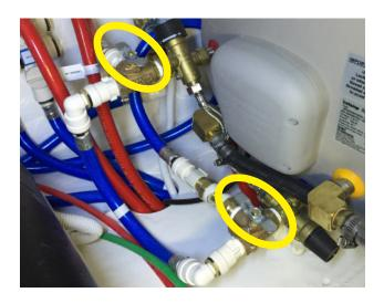
Figure 6-2: Water heater valves in normal operation position
