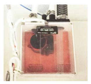
Figure 7-7: Graywater macerator drain box
