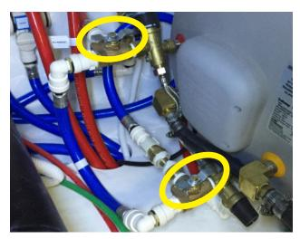
Figure 8-2: Water heater valves in bypass position
