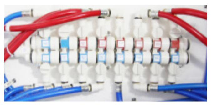
Figure 3-8: Fresh water system distribution manifold
