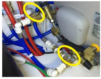
Figure 8-1: Water heater valves in normal operation position
