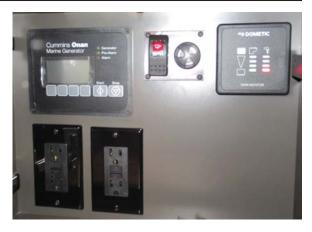
Generator control; high water alarm; holding tank monitor; and outlets, in the port companionway lower cabinet
