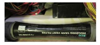
Tank vent air filter, behind access panel in head compartment
