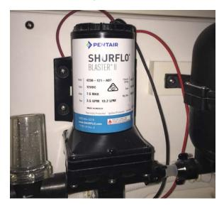
Raw water strainer (left) and pump, in the aft starboard mechanical space
