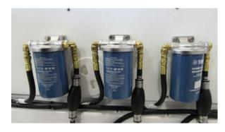
Gasoline fuel water separating filters (typical)
