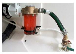
Air conditioning pump, strainer, and valve
