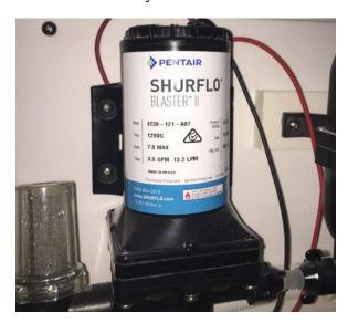
Typical raw water strainer (left) and pump
