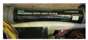
Tank vent filter, in the mechanical space near the holding tank
