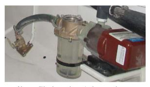
Air conditioning valve, strainer, and pump
