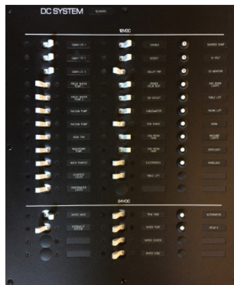
Figure 4-4: DC Distribution Panel
