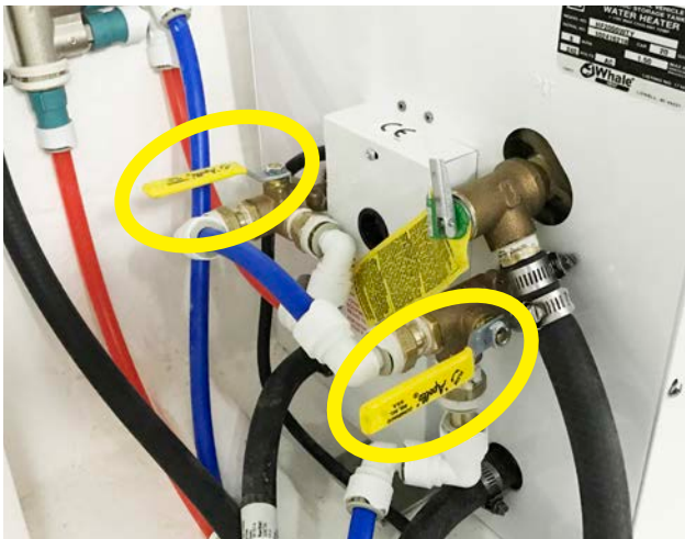
Figure 6-2: Water heater valves in normal operation position
