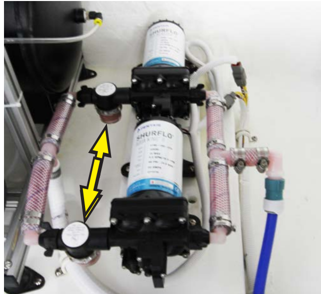
Figure 7-2: Fresh water pump and strainer (indicated by arrow)
