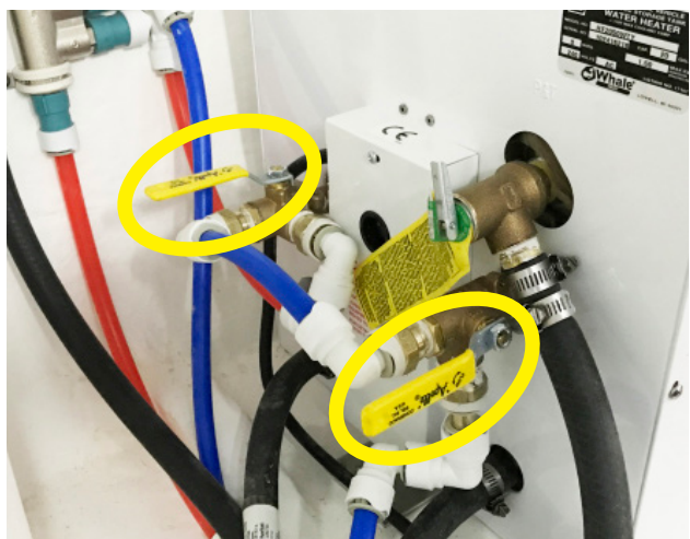
Figure 8-1: Water heater valves turned fully counterclockwise, in the normal operation position
