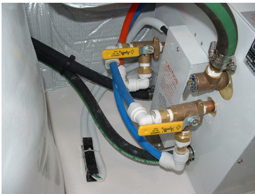
Figure 3-9: Water heater on port.
