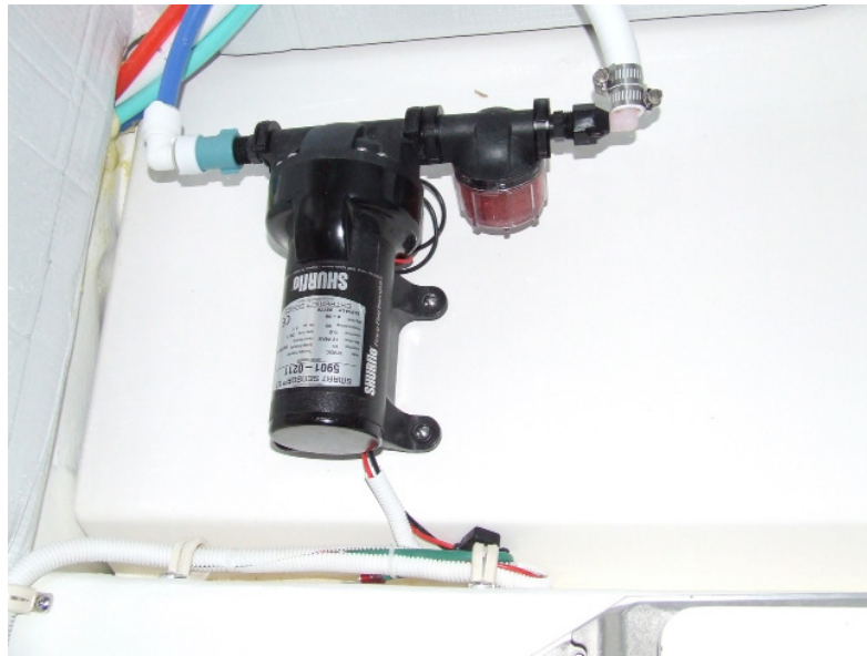
Figure 7-6: Fresh water filter and pump.
