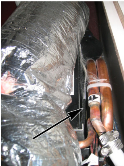
Figure 7-11: The A/C unit below the master stateroom aft berth storage. The arrow points to the mesh filter.
