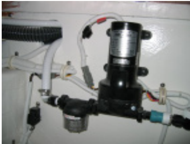
Figure 7-6: Fresh water filter and pump.
