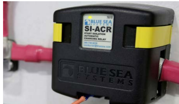
Automatic Charging Relay box (typical)
