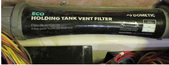
Tank vent filter (typical)
